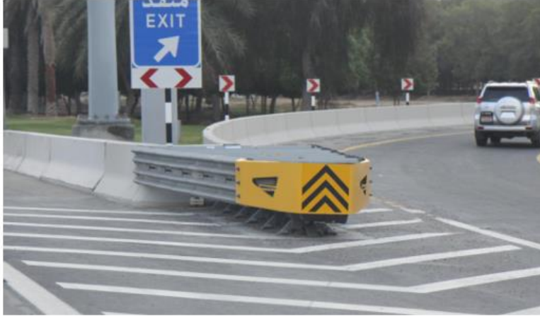
Figure 10.2 - Application of crash cushion at gore area
