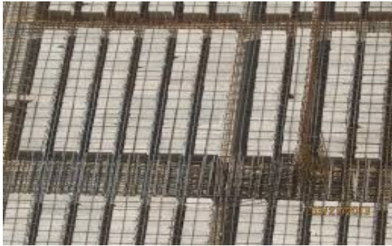
Figure 2.1: One way ribbed slab
